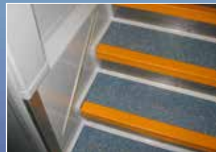
STAIR & STAIRWAY MARKINGS
